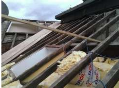
Old roof comes off and insulation goes in
