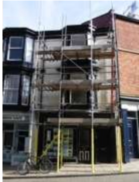
Scaffolding goes up
