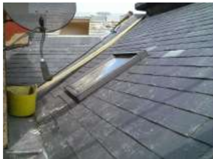
New roof in place
